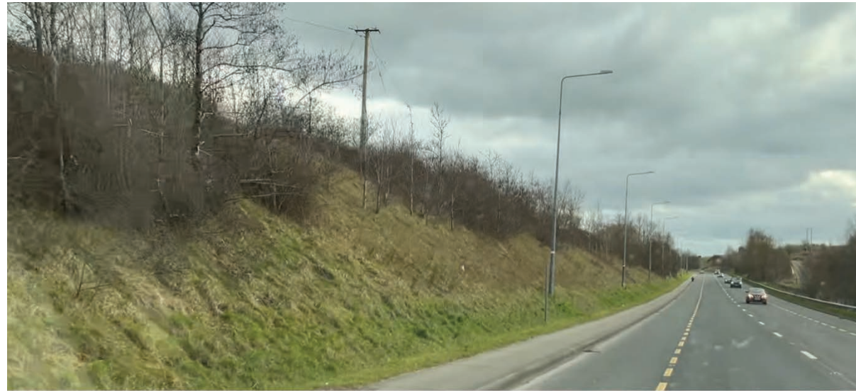
Figure 5.12 Image 5 View travelling South west along N85.
