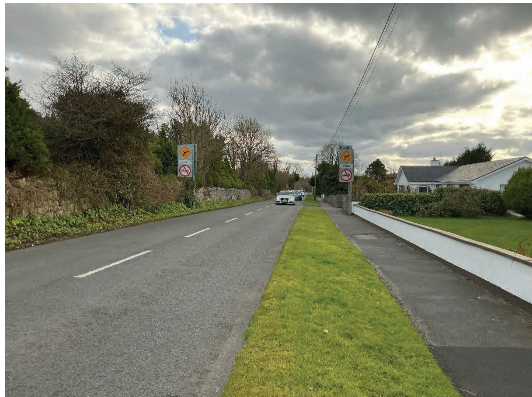
Figure 5.9 Image 2 View Travelling Southwest along R474
